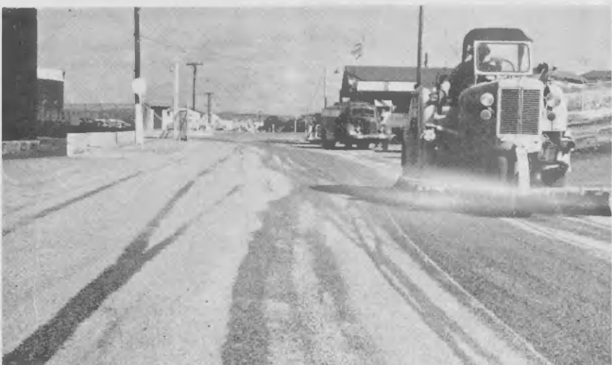
SEVERAL DAYS after the gravel has been spread and rolled, a road sweeper cleans excess material off the finished road. VARIOS DIA despues cu e graniet worde gespruit y plamá, un barridor di camina ta limpia e camina.
